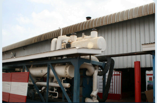
Industrial chiller installation
